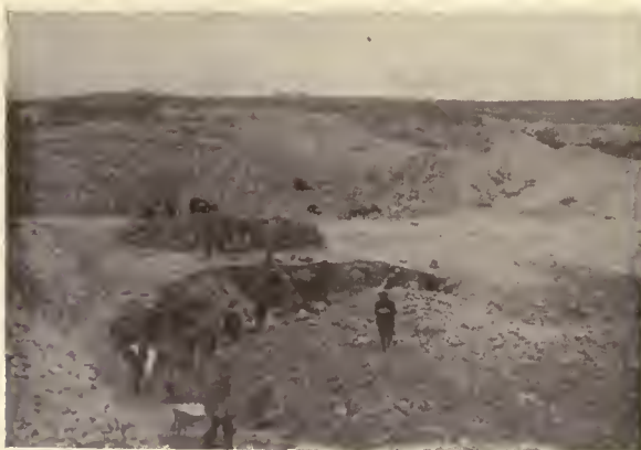
GETTING TO WORK ON THE FOUNDATION HOUSING BY STUDENTS AT PRAGUE
